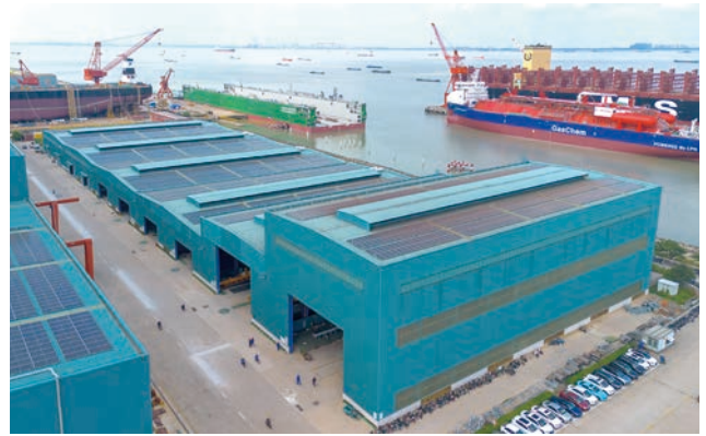
▲ 综合车间 (252m x 80m) Comprehensive Workshop (252m x 80m)
